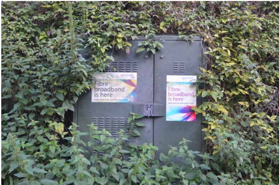
Figure 17: Most rural fibre broadband is currently delivered to cabinets with copper wires running to individual premises
